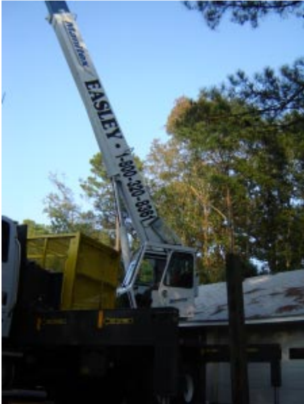
The 30-ton crane. It cost $913.60 to rent it.
