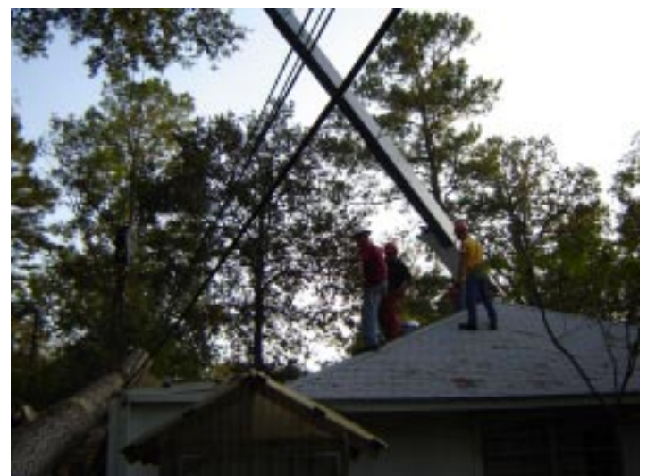
Clearing the power lines.
